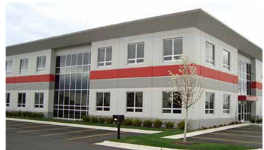
An example of a high quality office building using variations in building color, projections and windows to break up long walls.
